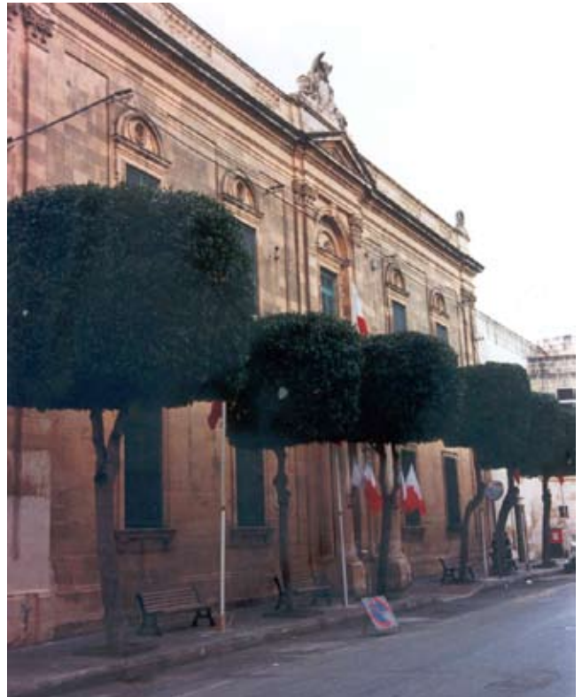
The premises that houses the Gozo Public Library, the National Archives/Gozo Section and Sir Arturo Mercieca Primary School at Vajringa Street Victoria
