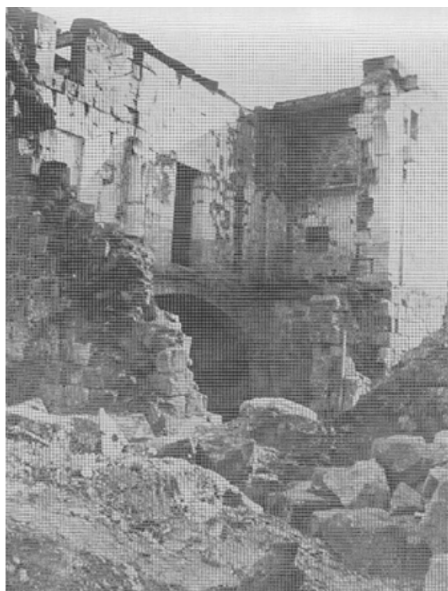
Building damaged by bombs in Mithna Street, Rabat, Gozo - 24.12.1941. Photo: C. Bezzina
