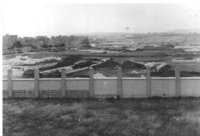
The laying of stone foundations at Tal-Hamri housing estate, Xewkija. C.1975
