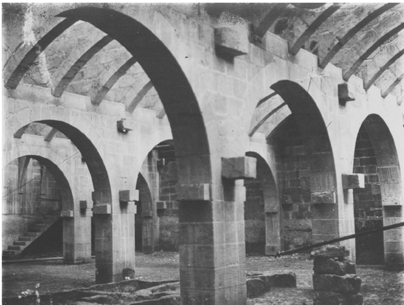
A late 1920's internal view of the reservoirs suggesting a likely reinstatement of the roofing slabs. Photo: Joseph Cremona died 24.I.1950 – © John Cremona
