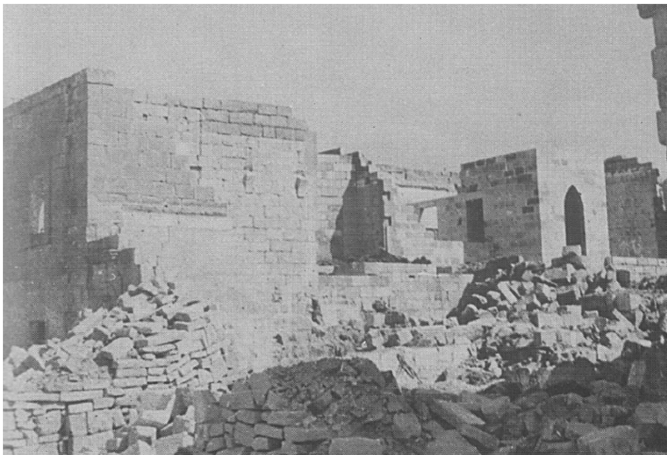
Houses damaged by bombs in Saguna Street, Sannat, Gozo - 10.10.1942. Photo: C. Bezzina
