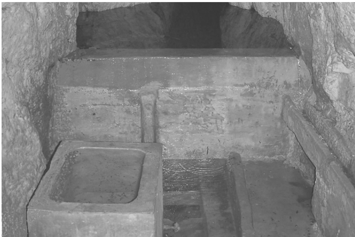
View of the 1840's water-collection gallery and settling-vats at Għar Ilma. Photo: Anthony Cauchi
