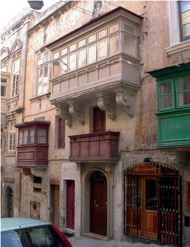
Figure 10.8. An example of a seventeenth century townhouse with open and closed timber balconies (G.A. Said-Zammit).
