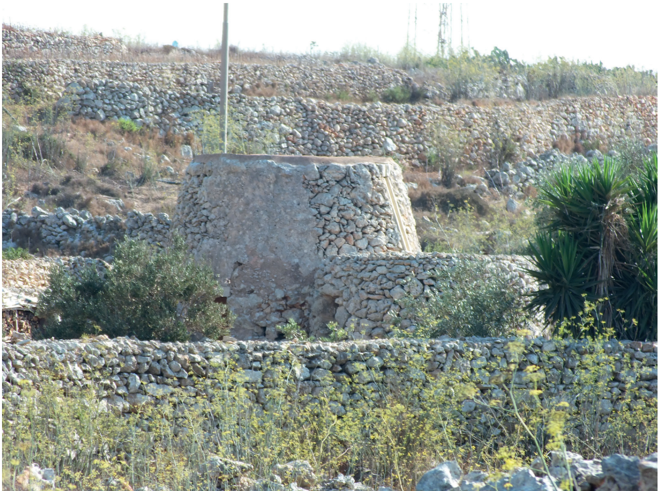
Figure 10.5. A girna integral with and surrounded by dry stone walling (G.A. Said-Zammit).
