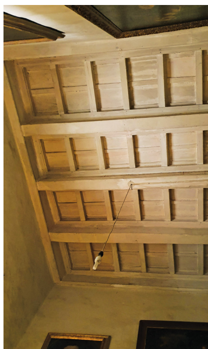
Above: coffered ceiling on the first floor Top right: view of garden from upstairs balcony
