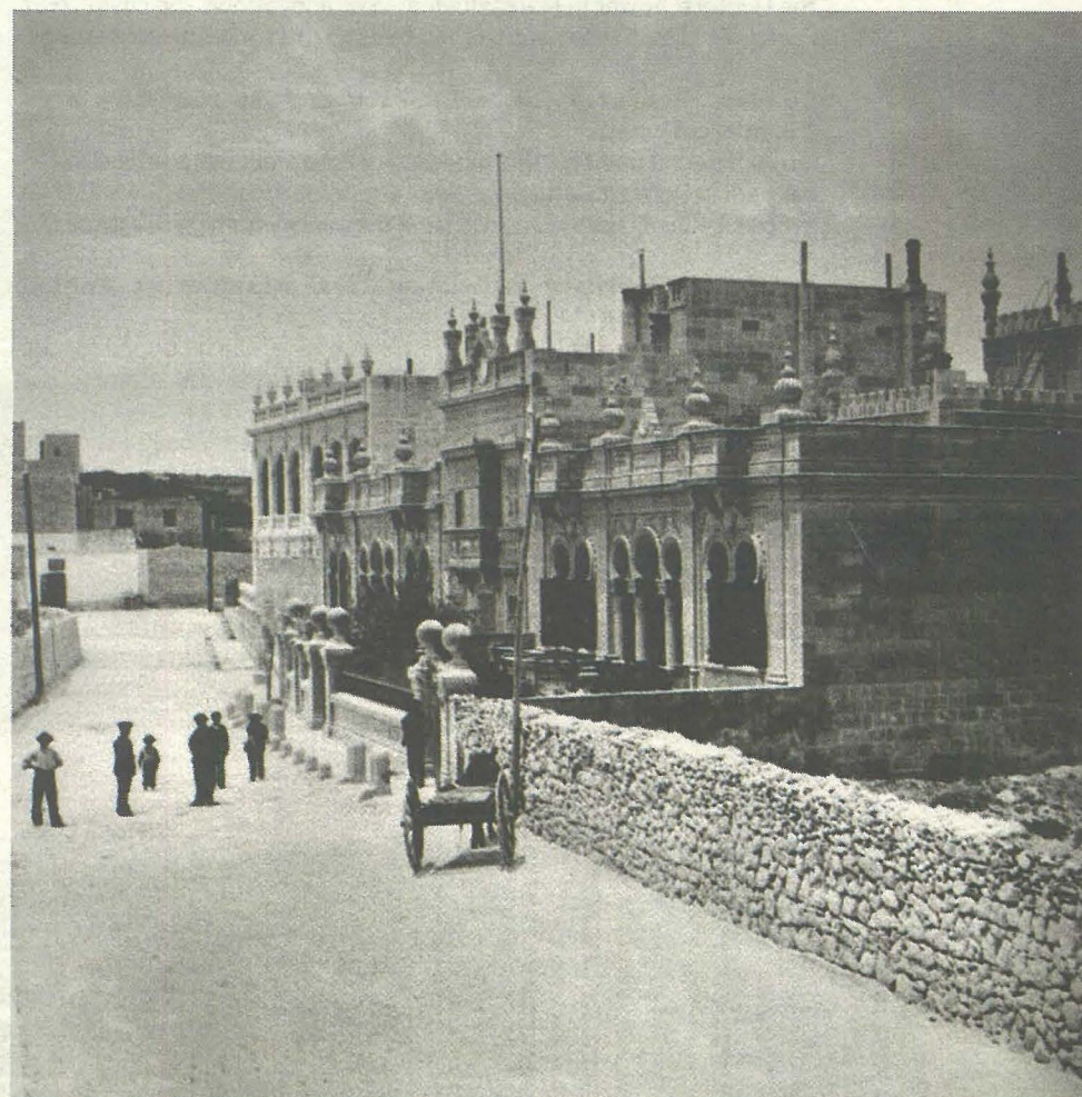
The Arabesque cluster of houses built by architect Emmanuele Luigi Galizia in Rudolph Street in the late Victorian times. PHOTO: RICHARD ELLIS
