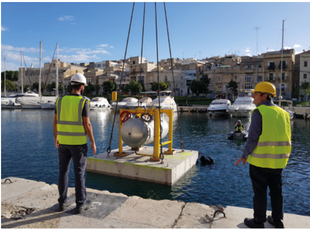
Daniel Buhagiar and Tonio Sant overseeing the deployment of FLASC at sea
