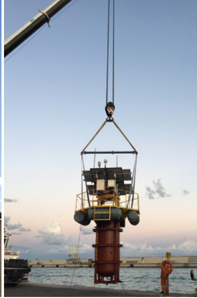
FLASC floater being lowered into the water for buoyancy tests at the Medserv quayside
