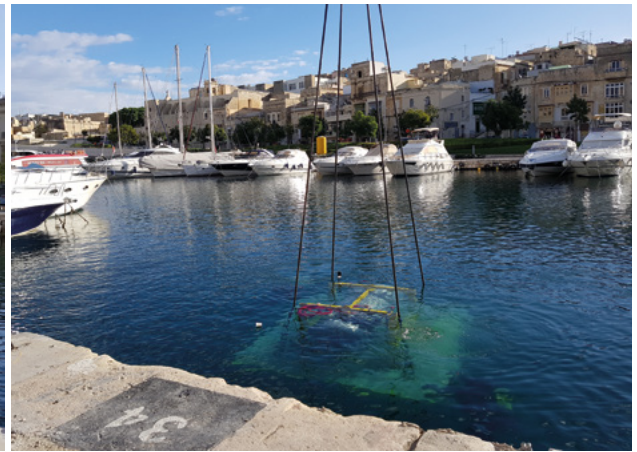
FLASC pressure vessel is successfully lowered into the sea
