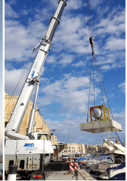
Medserv construction crane lifting the FLASC pressure vessel
