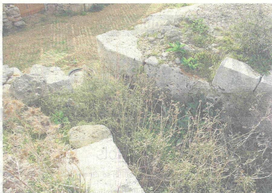
The borders of the embrasures consist of neatly cut ashlar masonry stones. In addition, one can also appreciate the thin layer of 'deffun' covering one of the 'merlons'.
