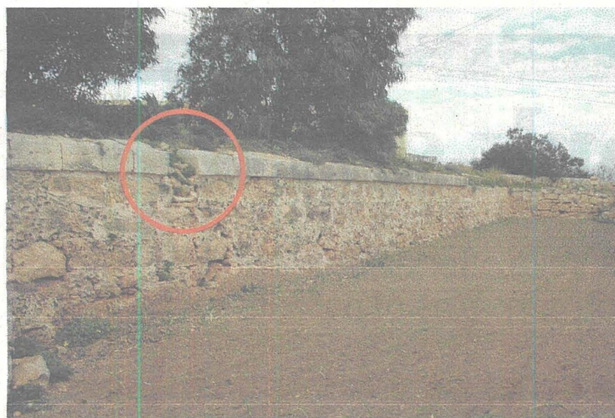
View of part of the flèche /redan and the short connecting wall. The red circle reveals the damaged water spout that drains the rain water from the upper part of the flèche , indicating that the soil and rubble infill was deposited there during the time of construction.
