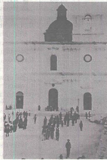
Fortunato Aguis, from Sliema, was nearly hit by stones thrown at him by an unknown woman who was helping in the construction of the Mellieħa parish church.
