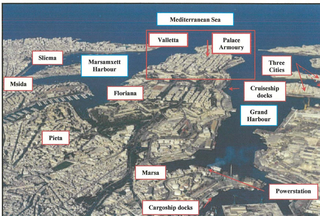
Figure 2-25 The coastal, urban and industrial regional environment of the Palace Armoury, Valletta 263
