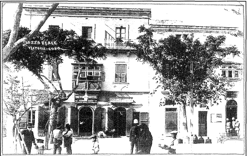
The Victoria Hotel, Piazza Reale, Victoria, Gozo, proprietor George Said, c. 1910. Real photograph.
