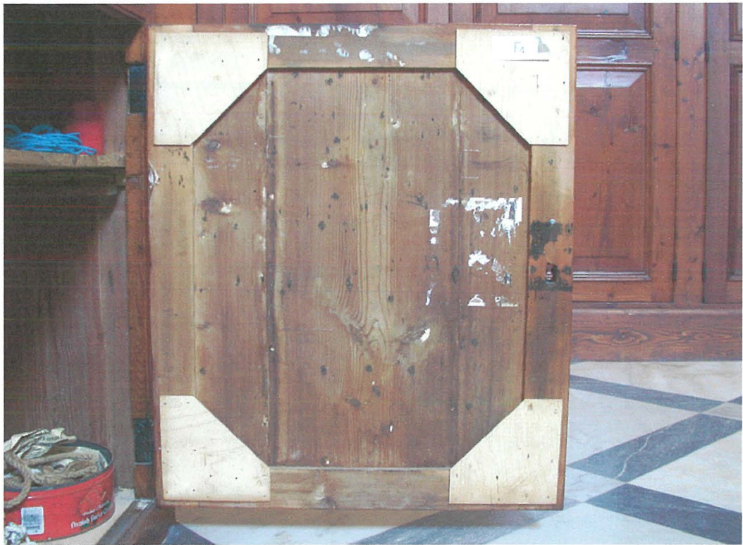
Plate 82 Pieces of plywood attached to support door – Stella Maris Church, Sliema
