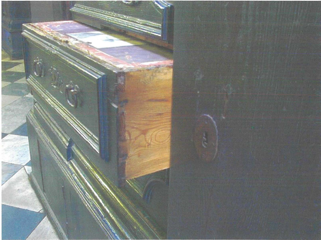
Plate 52 Dovetail joints used in drawer construction – St Paul’s Church, Valletta
