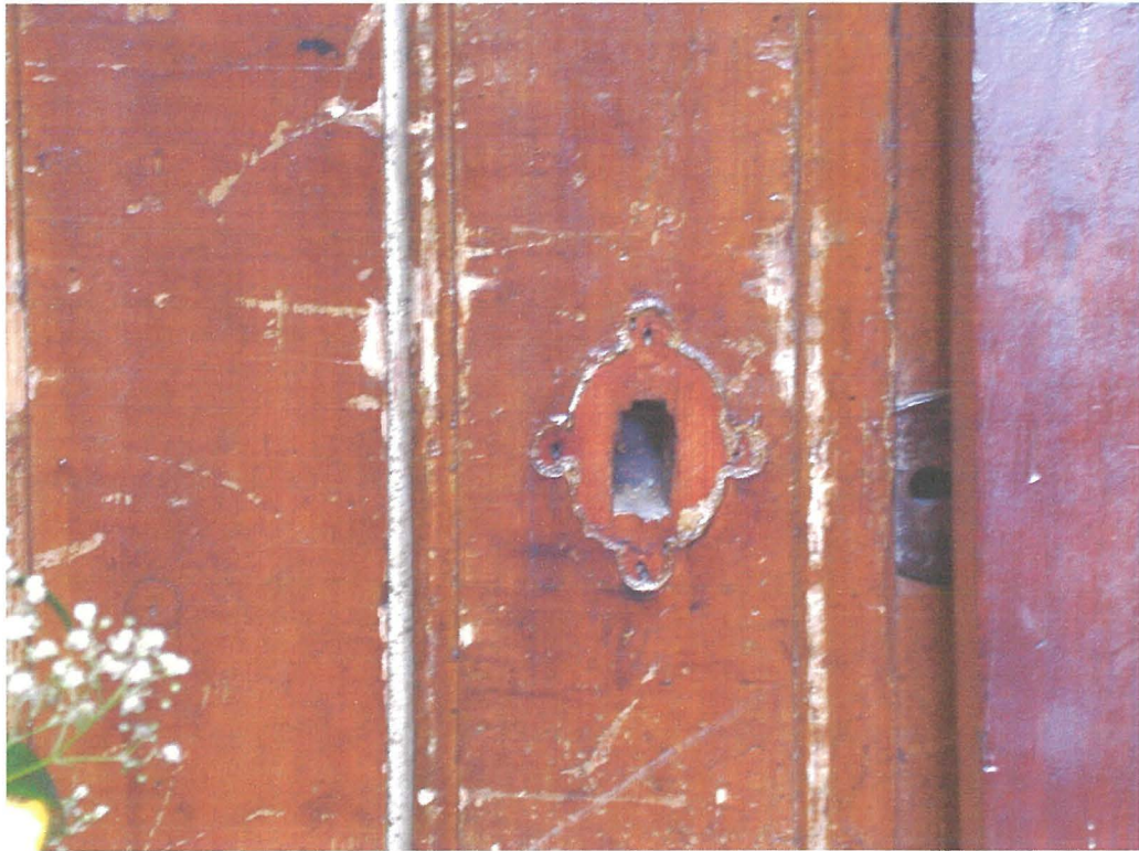
Plate 92 Abrasions and scratches on a door surface, new sacristy – St Helen’s Basilica, Birkirkara
