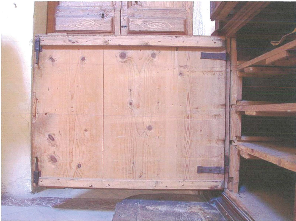
Plate 56 Door reinforced with horizontal nailed members – St Publius' Church, Rabat
