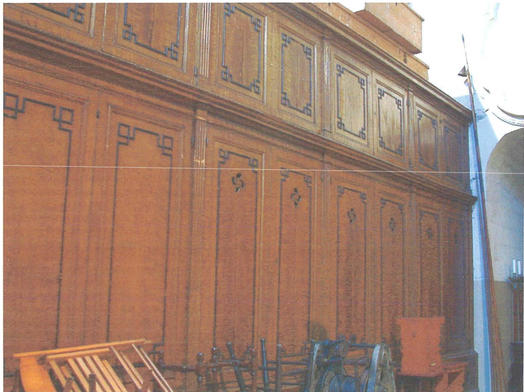
Plate 93 Chairs and benches close to furniture increasing the risk of damage, new sacristy – St Helen’s Basilica, Birkirkara
