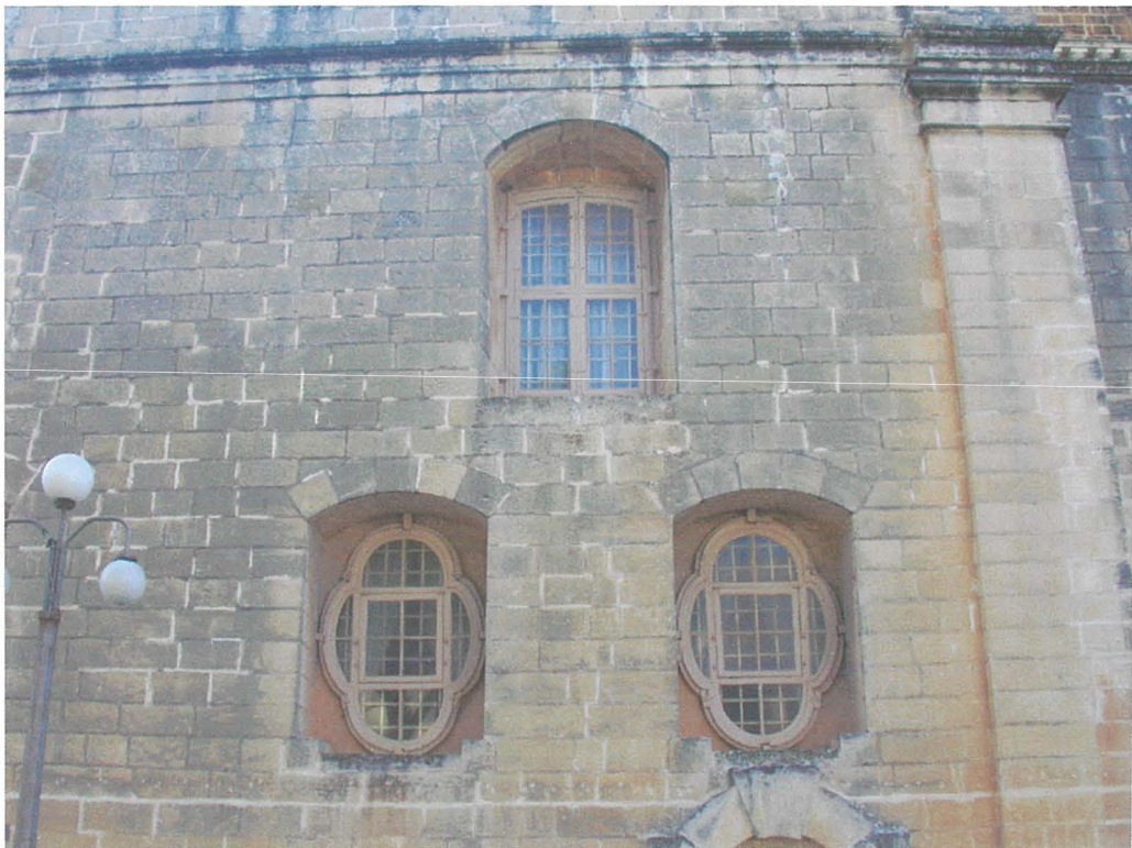
Plate 87 External wall of St Helen's Basilica old sacristy, Birkirkara
