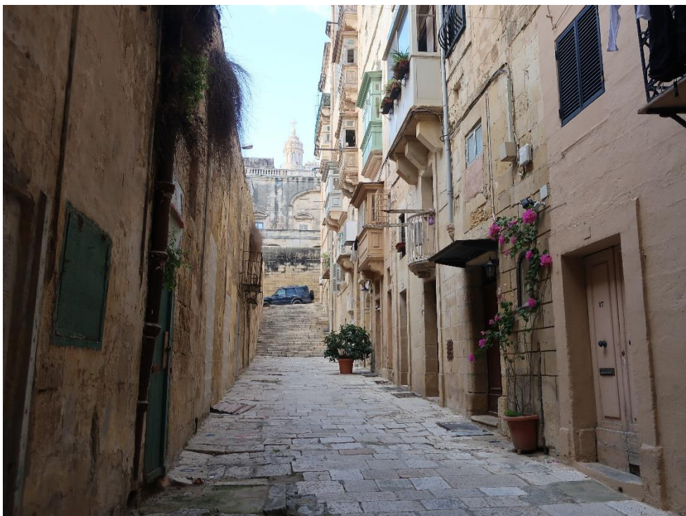
Figure 9 The building that will host the Valletta Design Cluster at il-Biċċerija
