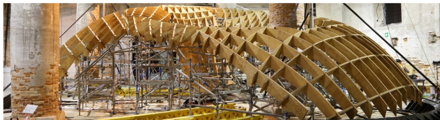
Figure 9 Falsework for the Armadillo vault, Venice Biennale, 2016, (Source: < http://www.armadillo-vault.com/armadillo-installation/ >)
