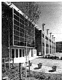
Figure 3.7: BRE office building itself in Watford (1995-1996). Source: www.lensebuildings.com/downloads/projects/05%20UK_BRE_Watford_LEnSE_Building_Report.pdf
