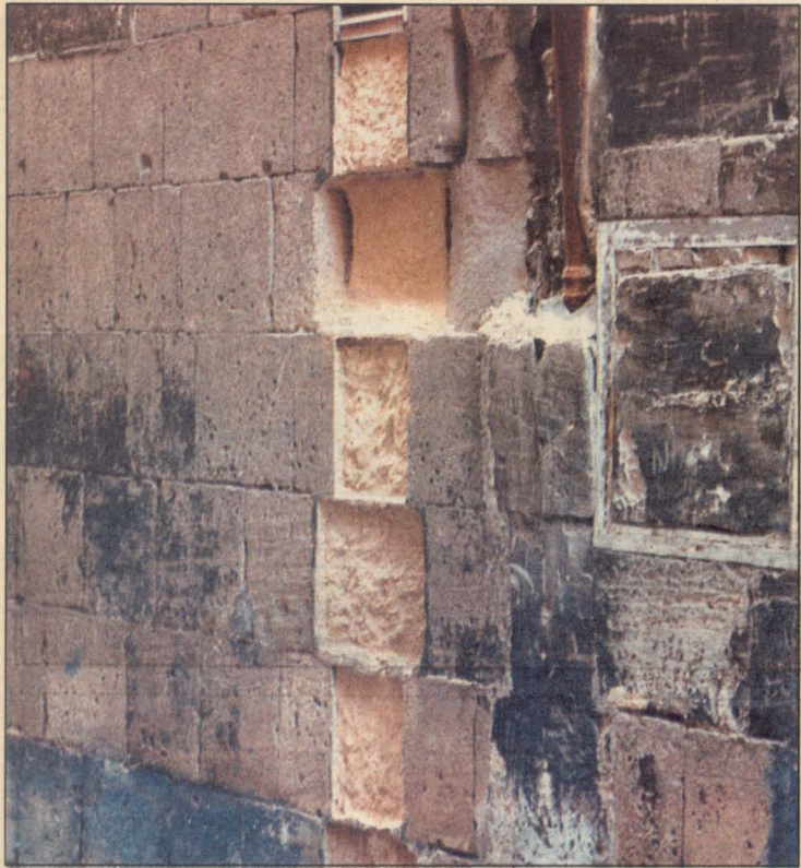
WEATHERING of poor quality dimension stone
