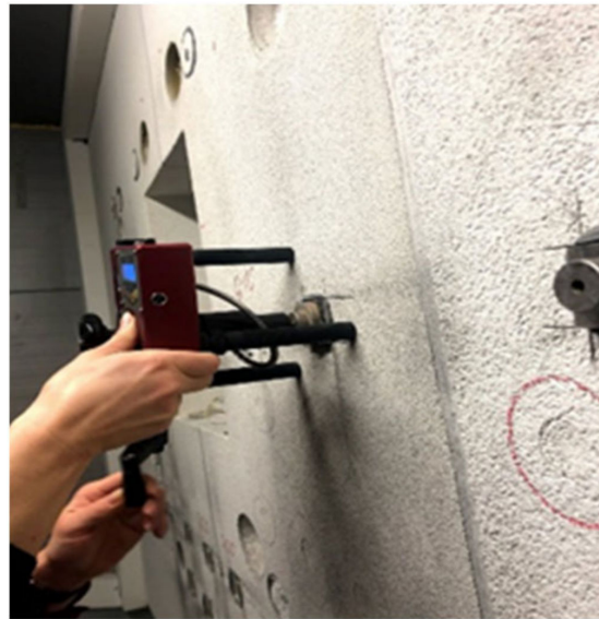
Figure 3. Testing of the bond strength of ETICS.
