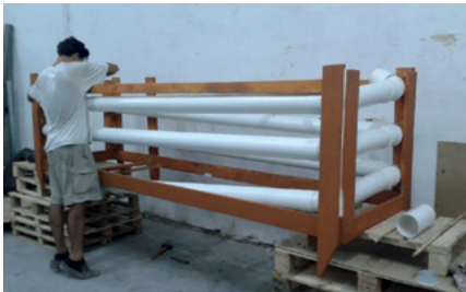
Figure 2.3: Construction of an eco-purifier for a very large pond
