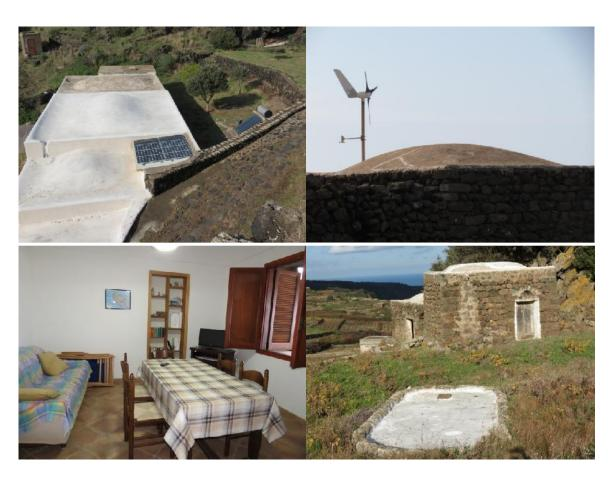
**Plate 4.1:** The dammuso, a typical dwelling on Pantelleria ideal to serve as an ecolodge due to the several environmentally-friendly and energy saving features, including the presence of a water cistern and its characteristic cupola. Photos: Karl Agius.
