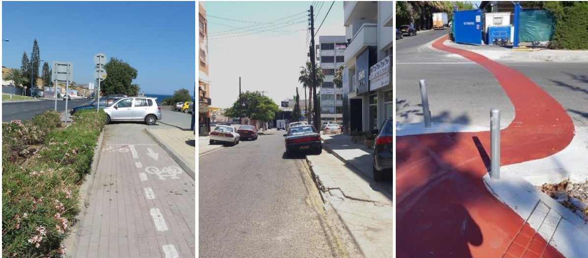
Figure 5.6: Negative examples of streetscapes in Limassol: abrupt end to cycling path, illegal parking on pavement, implementation of bicycle lanes gone wrong (left and middle photos by author; right photo: Hadjiioannou, 2019)
