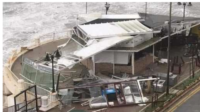
Figure 6: Coastal structures damaged by the storm on the 24 th February 2019. Source: Times of Malta
