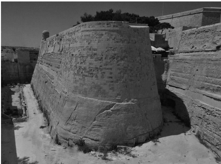
2: View of St. James Bastion with its rounded orecchione, one of the four bulwarks along Valletta's land front enceinte; St James Cavalier is visible in the background, right (Image source: Stephen C. Spiteri).
