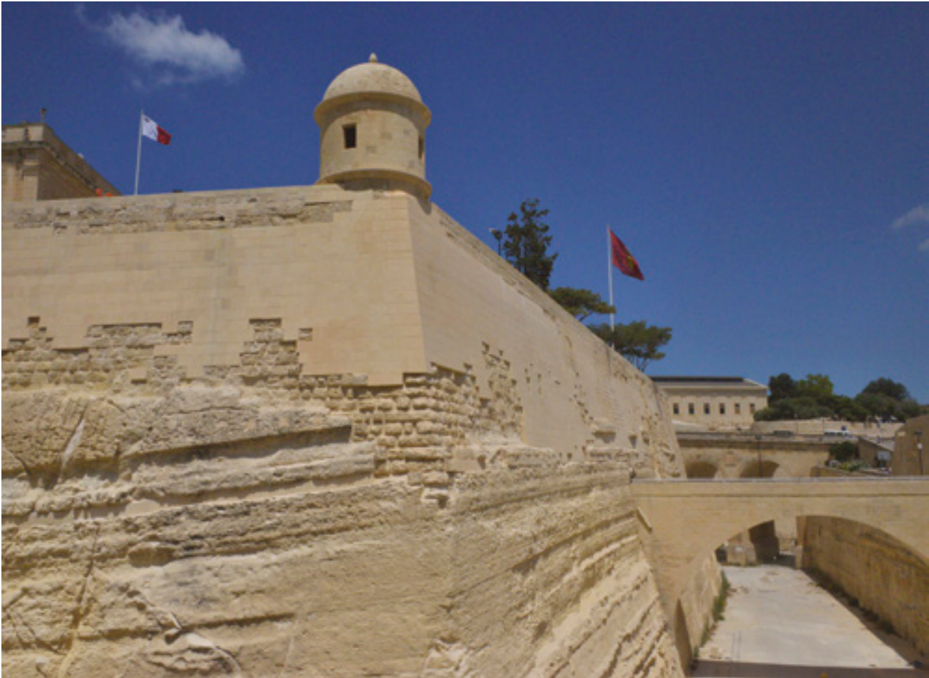
Rock hewn bastion and ditch of the landfront fortifications of Valletta.
