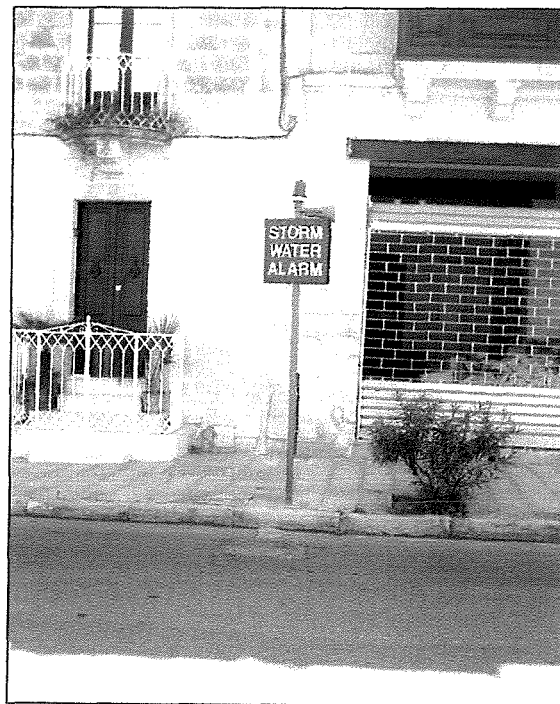
Plate 5.16: B'Kara Storm Water Alarm
