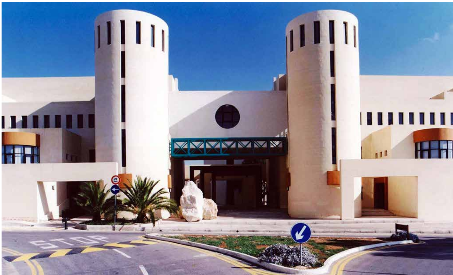
Fig. 30: Gateway building referred to as Mikiel Anton Vassalli building (photograph credit: Richard England) Overleaf – Figs. 31 and 32: Mikiel Anton Vassalli building
