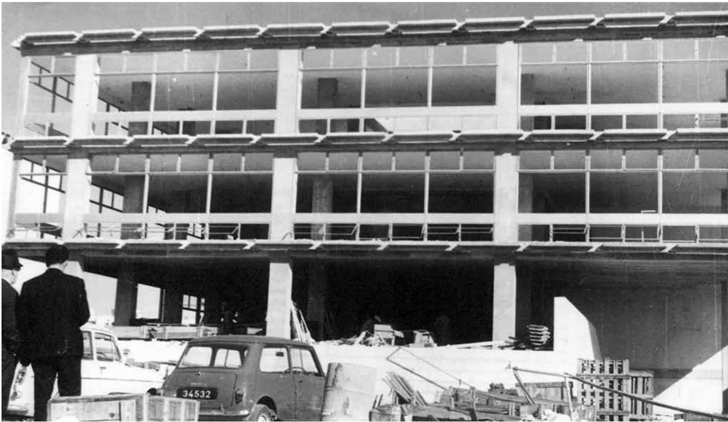
Fig. 9: The Library building under construction
