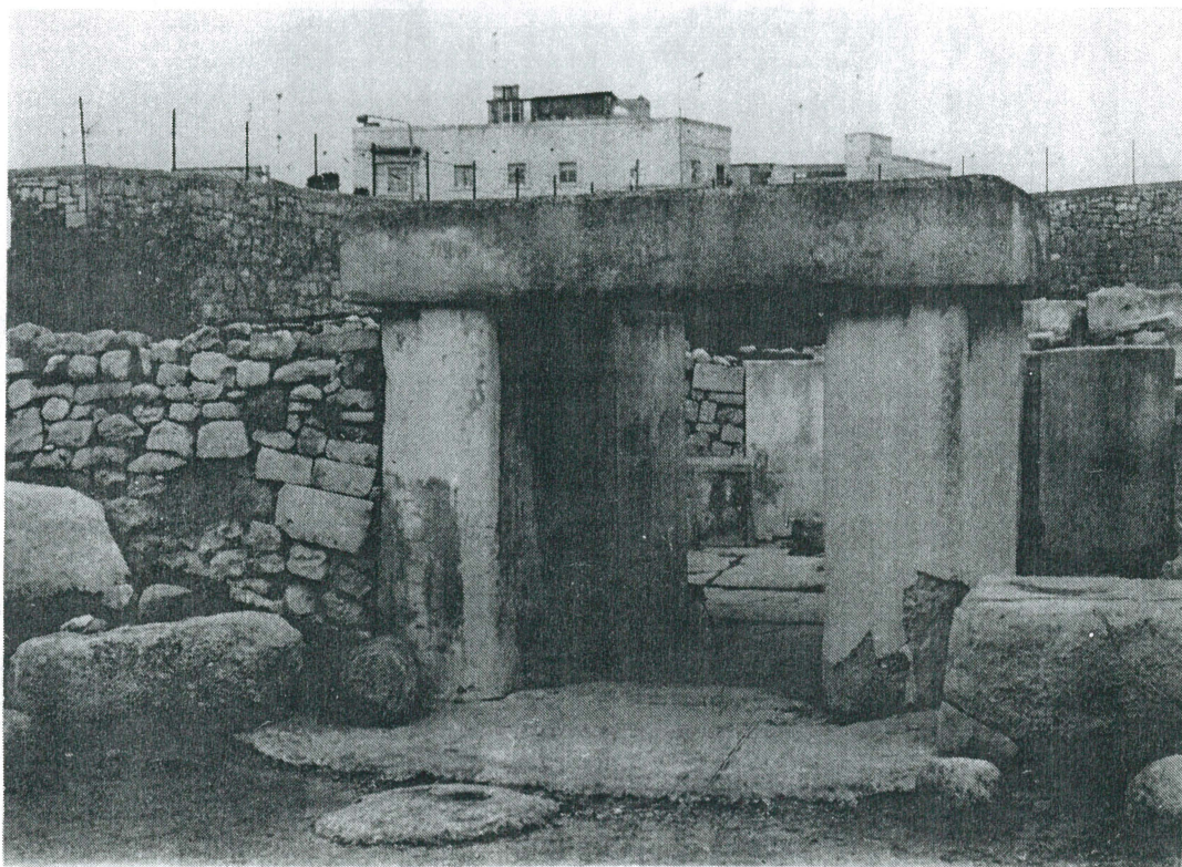
Plate 6 Main doorway of the Tarxien Temple Complex, restored in concrete.
