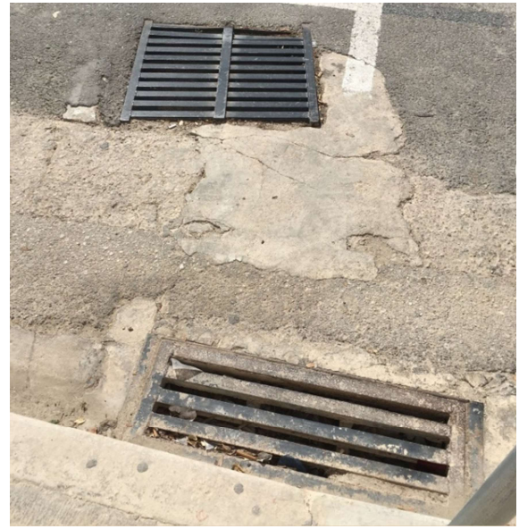
Figure 92: Basic or sporadic gutters/gratings observed in a civic square (left) and street (right). In the case of the gutter the water is discharged into to street carriageway which then has no gratings.
