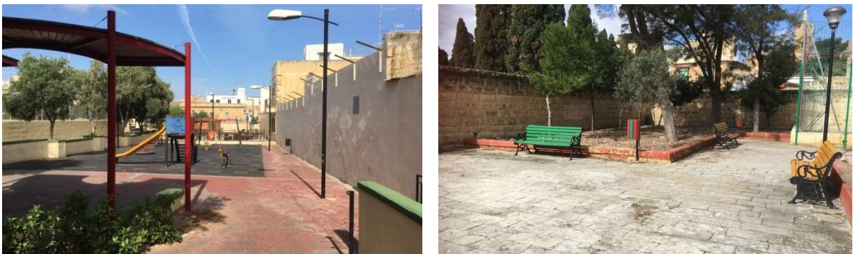
Figure 41: Images showing a bad transition between a public and private space creating blank walls (Tarxien and Pietà)
