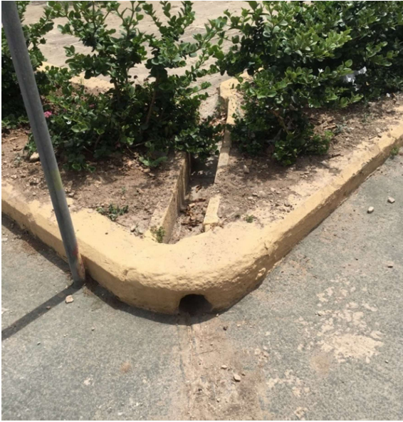
Figure 92: Basic or sporadic gutters/gratings observed in a civic square (left) and street (right). In the case of the gutter the water is discharged into to street carriageway which then has no gratings.
