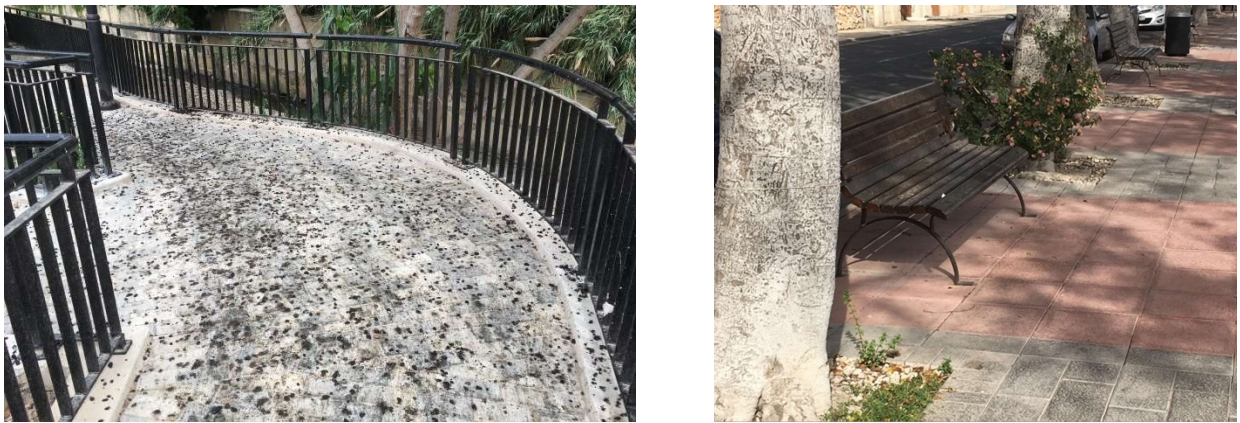
Figure 104: Images illustrating how trees created nuisance, firstly due to dirty and slippery paving, secondly due to benches littered with bird droppings
