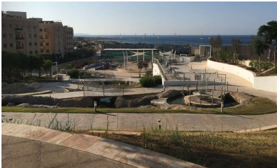
Figure 119: The ramped footpath which informed the garden's layout due to the site's topography (Pembroke)
