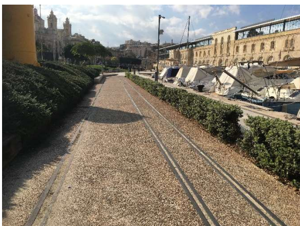
Figure 114: Historic artefacts (rails, stone slabs and ship bollards) retained and incorporated in the design
