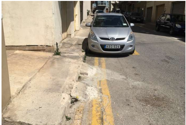
Figure 76: Images showing poor provision for pedestrians. Infrastructure is either uneven or minimal.
