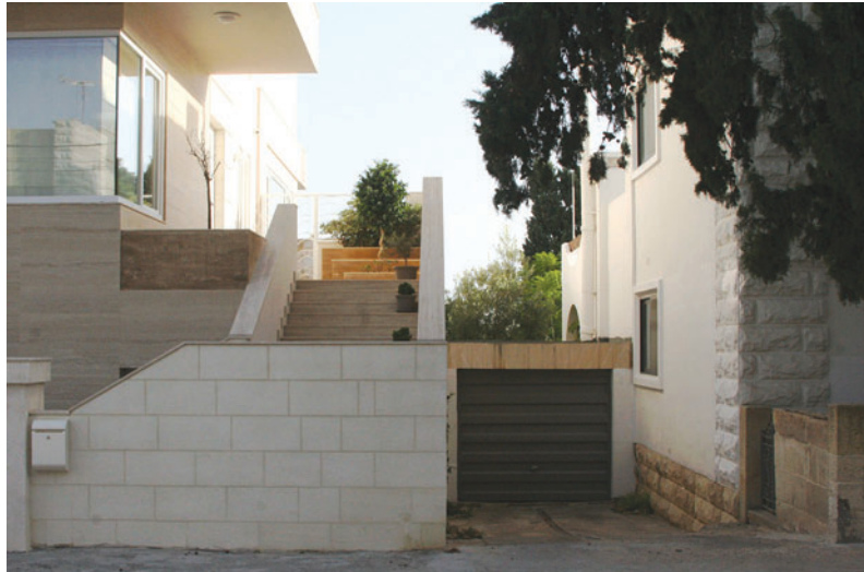
Figure 36: Garage within the side curtilage
