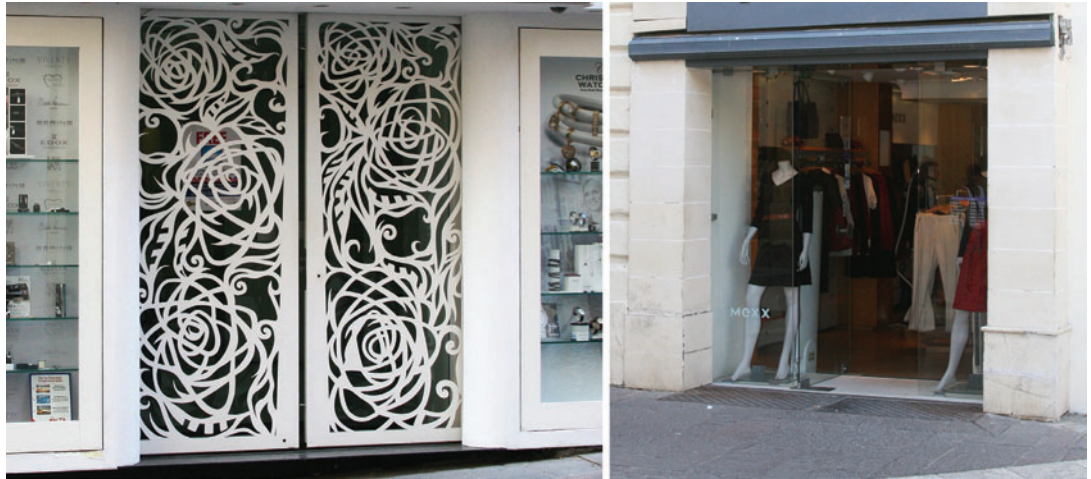
Figure 78: Well-designed (left) and poorly detailed (right) shop front security shutters
