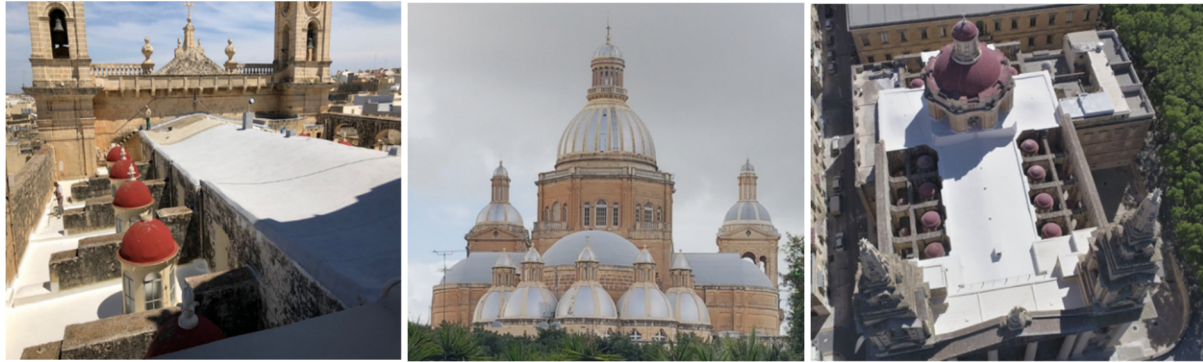
Figure 2. Initiatives and examples of cool roofs. (Left): The Collegiate Archmatrix Parish Church of Saint George, Qormi (Malta). (Mid): The Basilica of Christ the King, Paola Parish Church (Malta). (Right): The Saint Publius Parish Church, Floriana (Malta). Photographs by author RCV (2018–2020).
