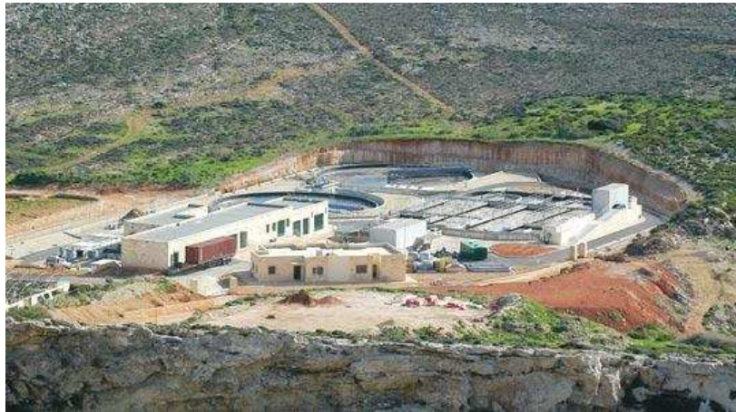
Figure 5: Iċ-Ċumnija Sewage Treatment Plant, Anchor Bay, Malta (Source: http://www.timesofmalta.com )
