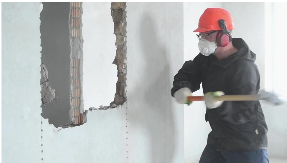
Figure 1: Removing bricks from a wall in a construction site (Source: pond5.com)
