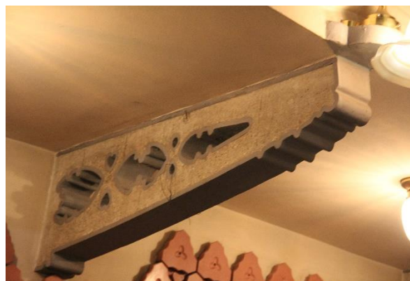
Fig. 2: Concrete cantilever supporting the balconies in Petőfi Theatre in Veszprem (1908)
