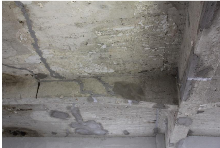
Fig. 3: Industrial building (1930) in Budapest refurbished to offices
