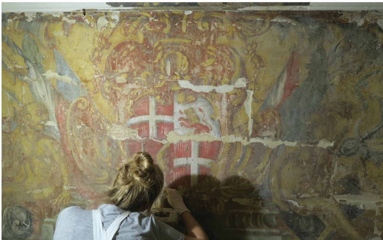
A conservator at work cleaning the painted frieze at the Chapel of Palazzo de La Salle, Valletta. Photo courtesy of the Department of Conservation and Built Heritage
