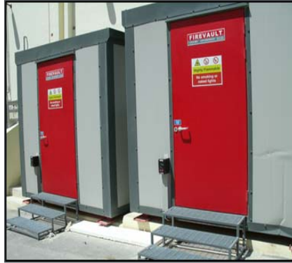
Laboratory Chemical Storage Areas with integrated Spill Containment
