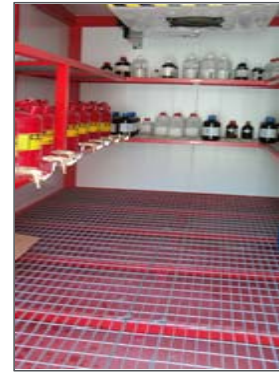
Laboratory Chemical Storage Areas with integrated Spill Containment
