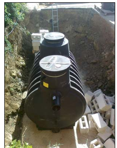
Installation of an Oil Water Interceptor in the Employees' Car Park
